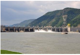
Dam of the Iron Gates - Serbia - Rumania
